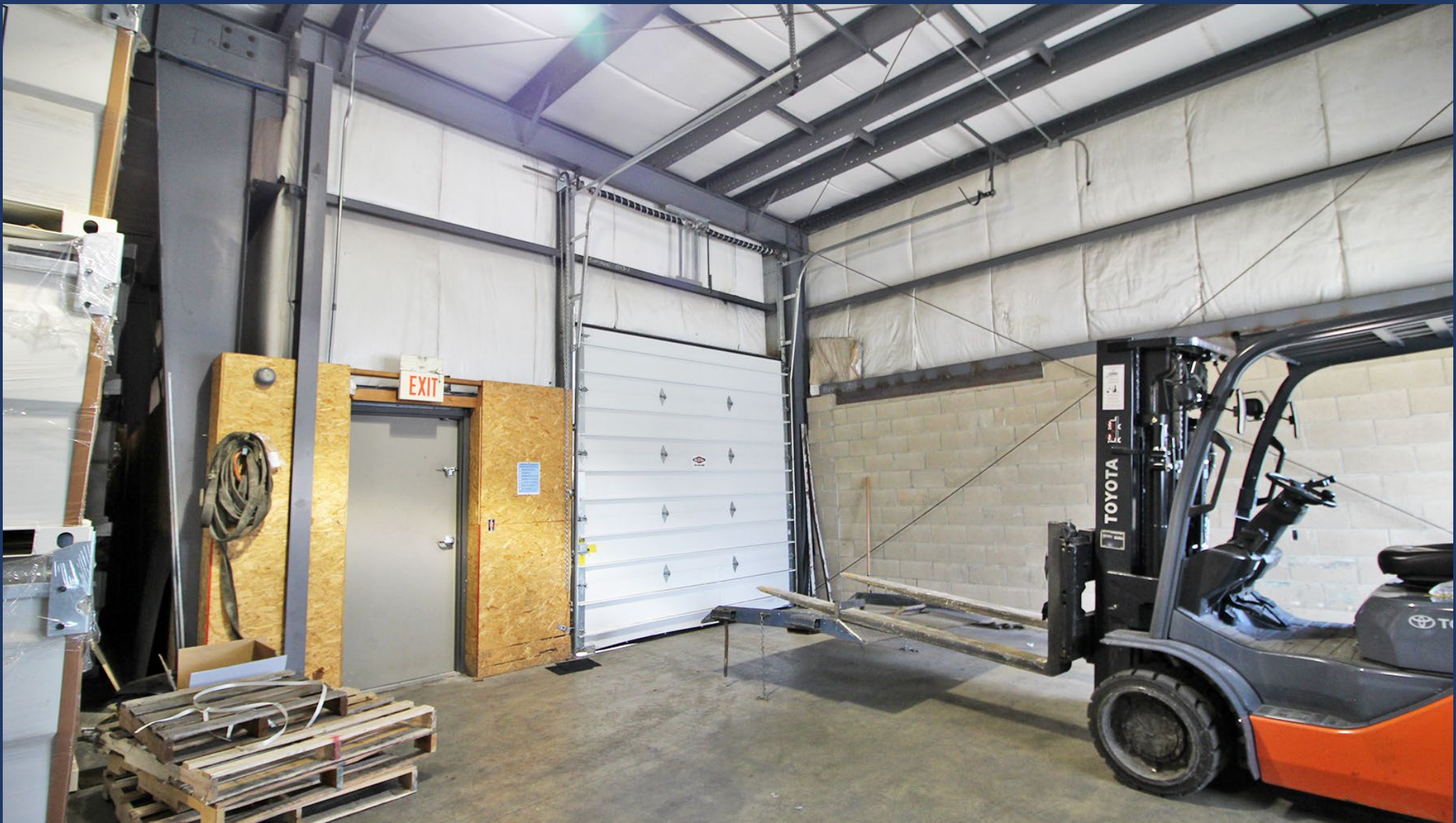
One Loading Dock
